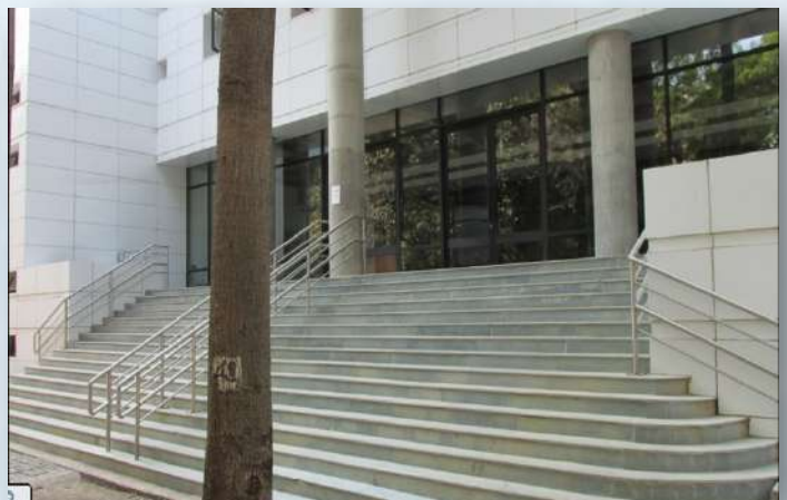
New CSE Building
