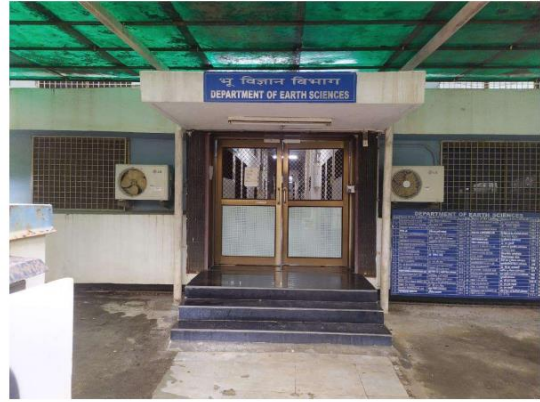
DEPARTMENT BACK GATE
