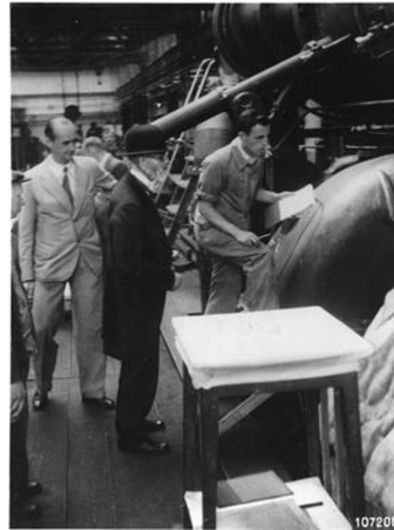
Commissioning of world's first industrial gas turbine, Neuchatel, 1939 (Stodola at age 80)
